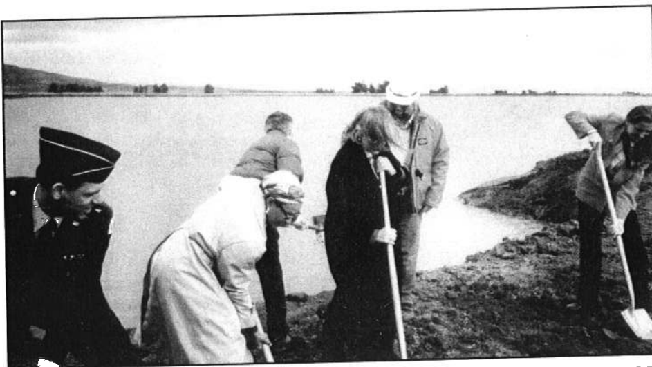
Breaking dyke to allow Bay waters into Sonoma Baylands, from left, USCOE District Engineer Col. Richard Thompson, State Sen. Barbara Lee, Rep. Lynn Woolsey (D-Marin) and White House environmental advisor Katy McGinty
